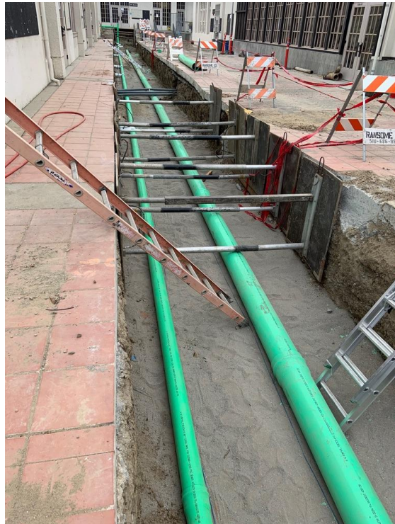
Storm drain replacement and rerouting under the PHS breezeway.
