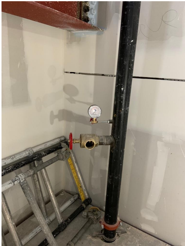
High pressure fire line that feeds the fire sprinkler system (left), and duct work at the elevator shaft (right).
