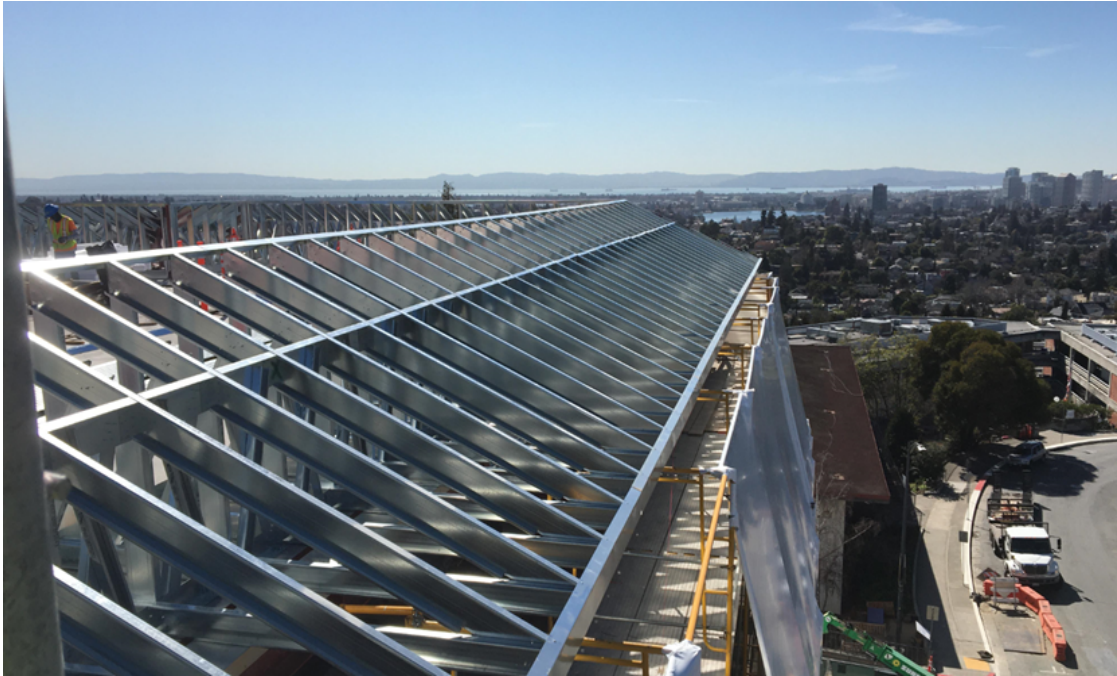
Installation of mansard roof.
