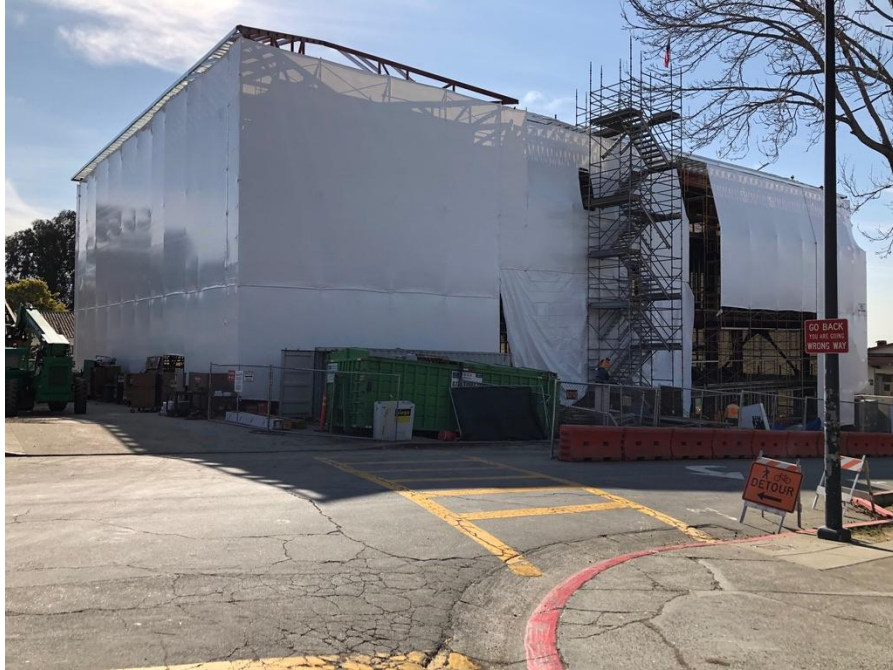
Shrink-wrapping of the STEAM building exterior to protect interior work from rainy weather.
