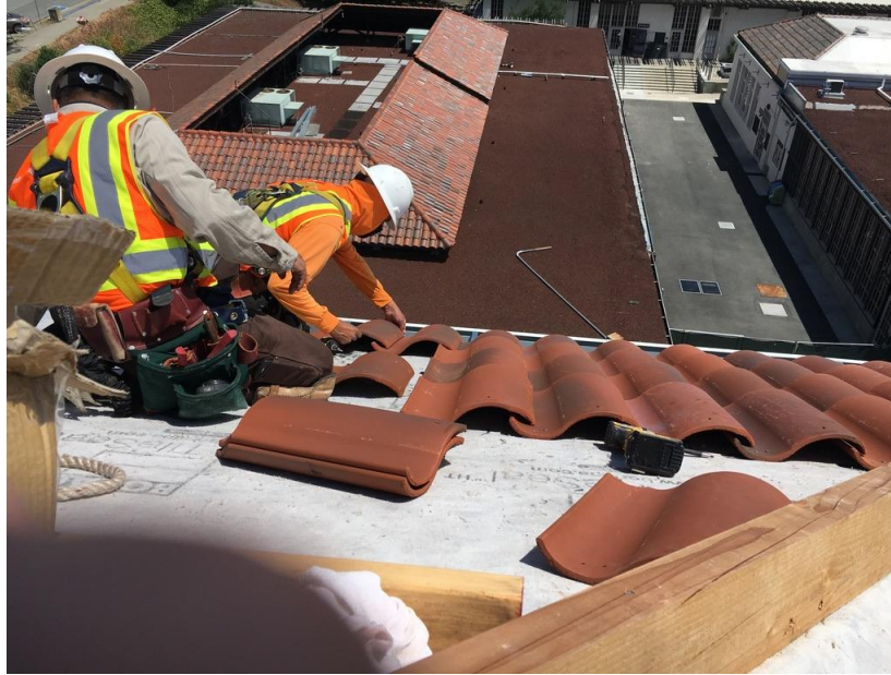
Installation of clay tile on mansard, with view of the PHS breezeway and 30s building at right.
