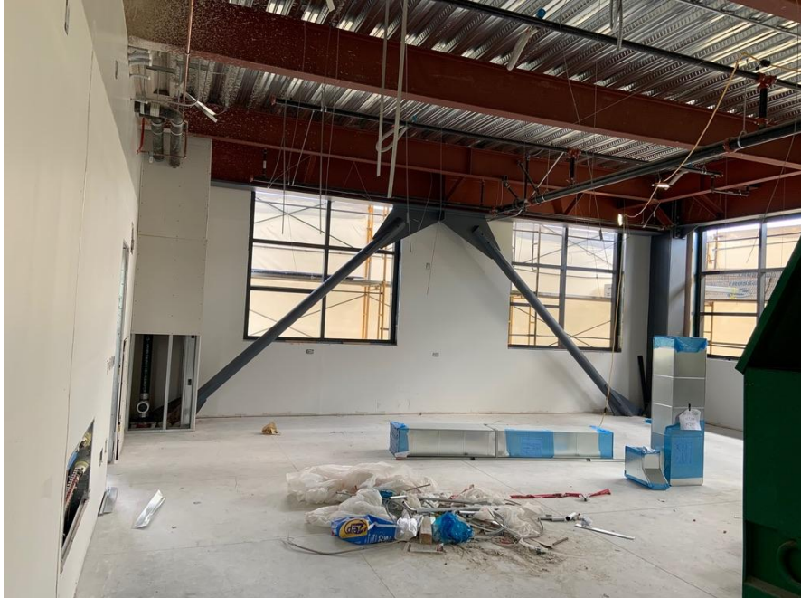
Installation of ductwork in science classrooms.
