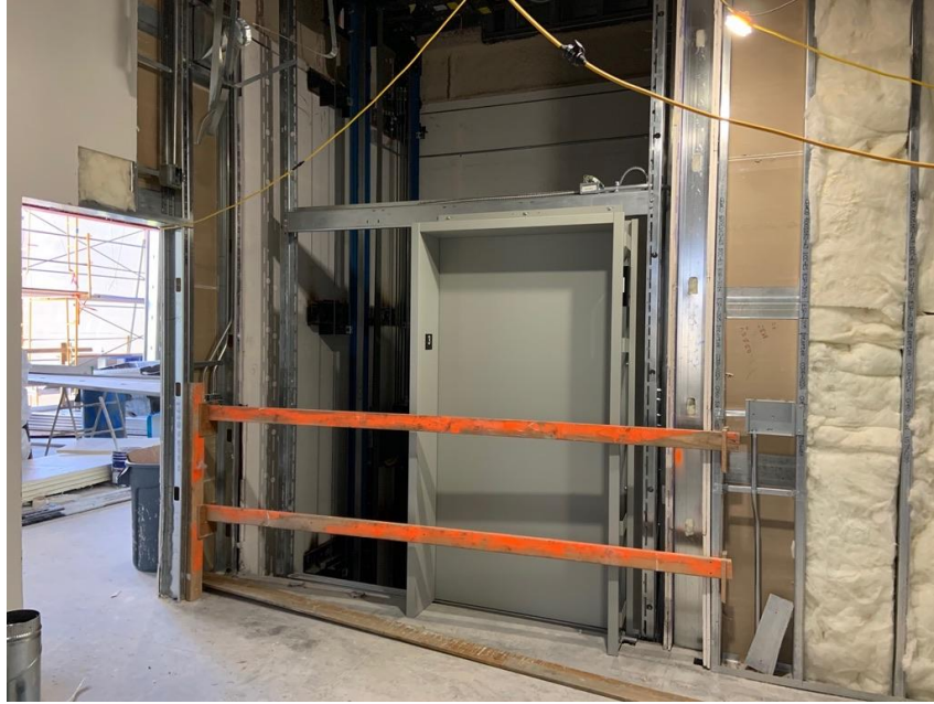
Installation of the elevator.
