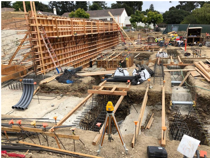
Placement of structural rebar in the footings and forms for pouring a concrete retaining wall.
