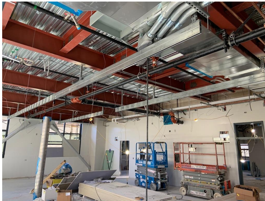
Infrastructure for flexible, movable power lines for student workstations.
