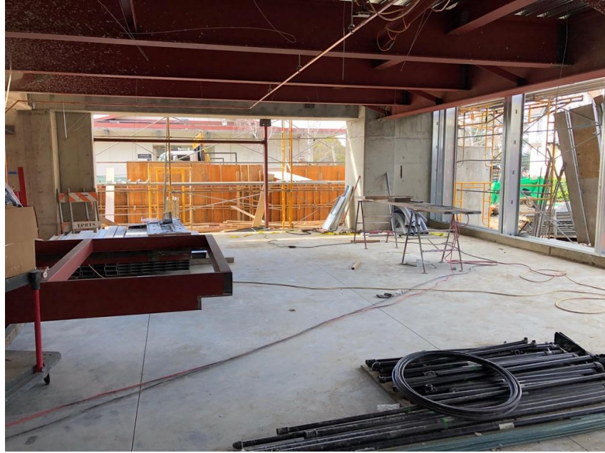
Poured concrete walls and completed slab on grade for the new 2D art room.
