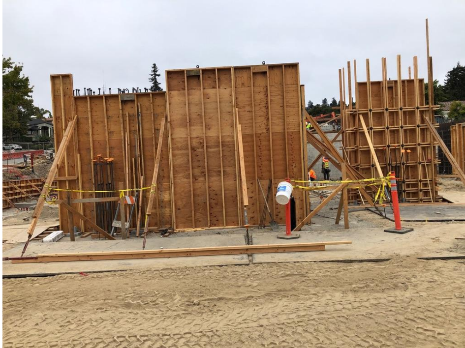
Forms for pouring a concrete wall at the future site of the art patios.
