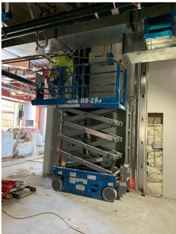
High pressure fire line that feeds the fire sprinkler system (left), and duct work at the elevator shaft (right).
