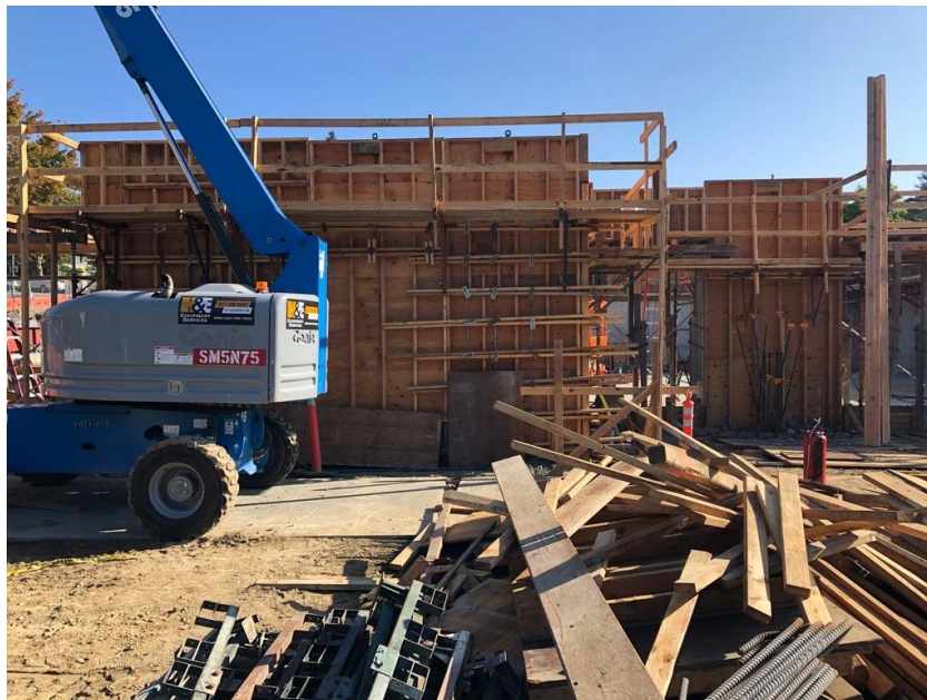
Completed forms ready for the concrete pour.
