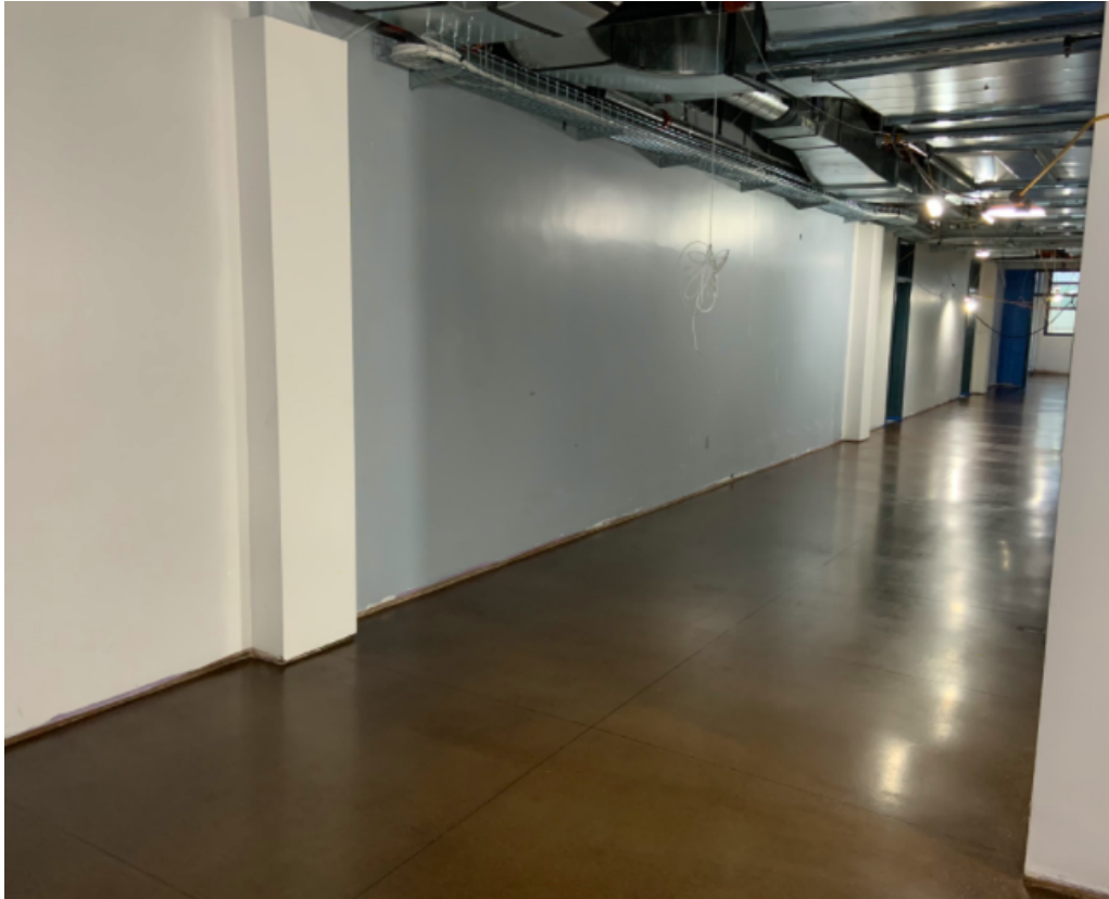
STEAM building hallway with stained and polished concrete floors.
