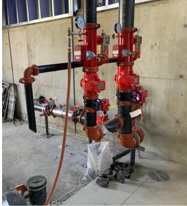
Riser assembly for the Performing Arts Center's fire sprinkler system.
