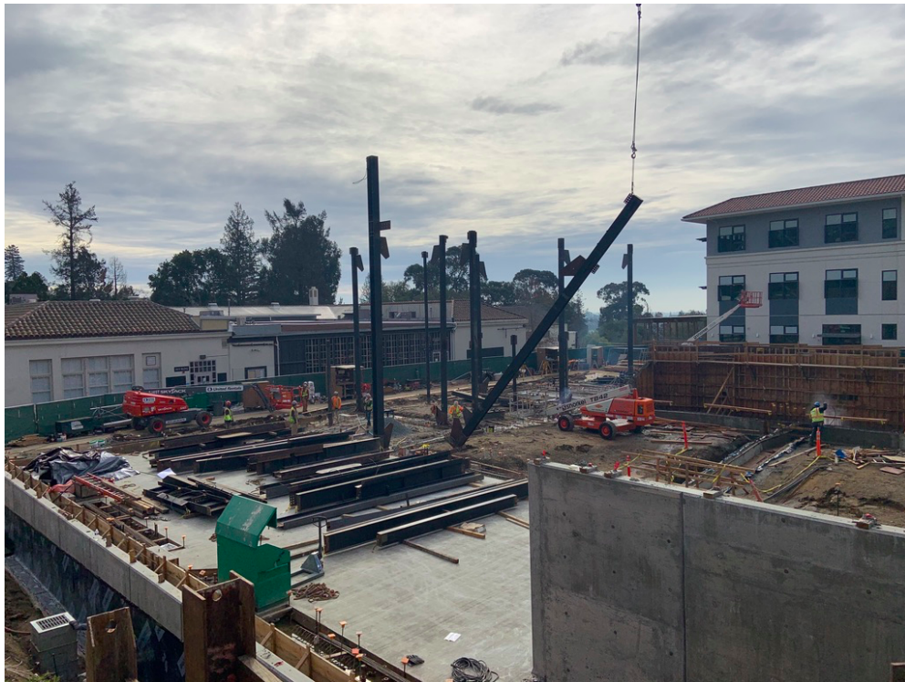
Setting the steel columns in the completed foundation for the Performing Arts Center, with a view of the completed STEAM building.
