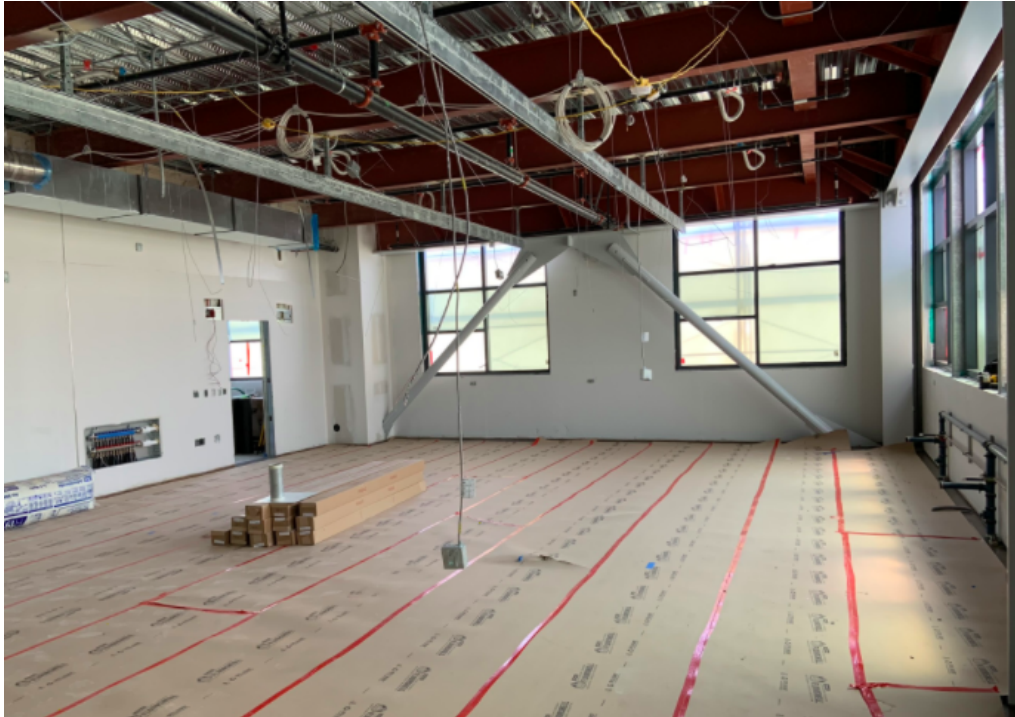
STEAM building classroom featuring exposed steel brace frames.
