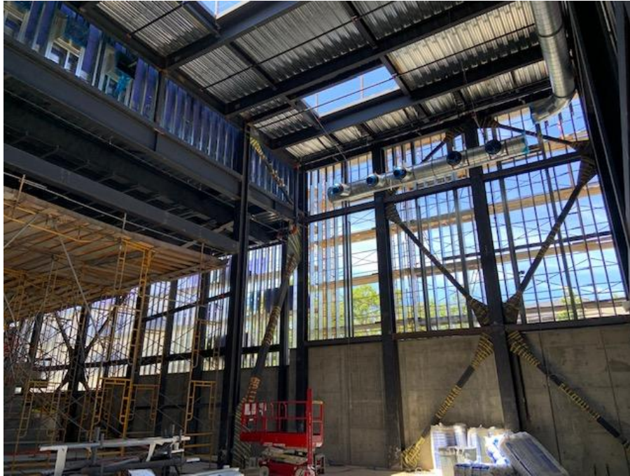
Metal stud framing and seismic steel brace frames in the Performing Arts Center. Also shown are the pan deck ceiling of the high stage roof and smoke hatches required for fire safety.
