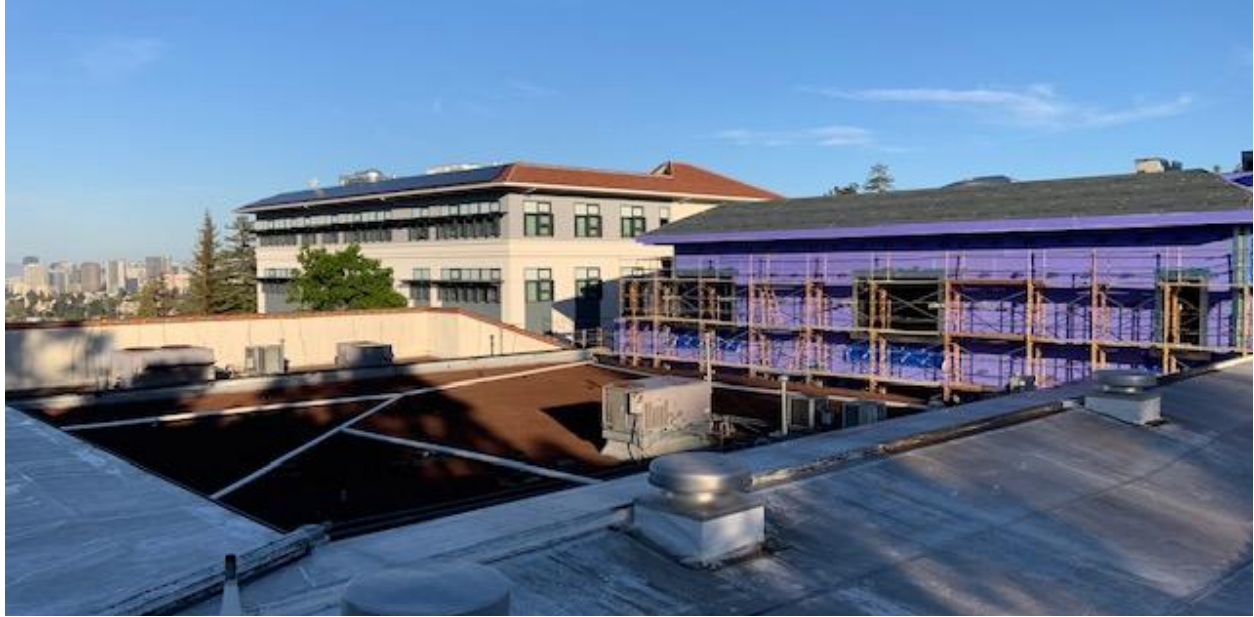
View from the 30s building roof showing installation of dens glass sheeting on the Performing Arts Center exterior, prior to application of stucco.
