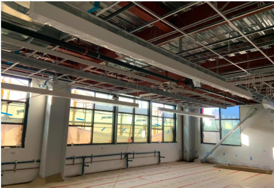
STEAM science lab with plumbing for acid waste drainage system.
