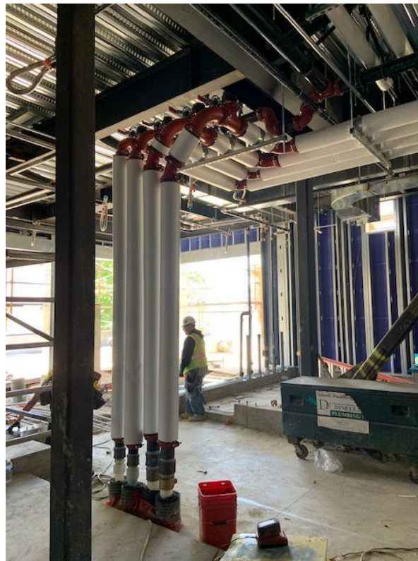
Hydronic system for piping hot and cold water to the Performing Arts Center from the STEAM building's rooftop HVAC system.
