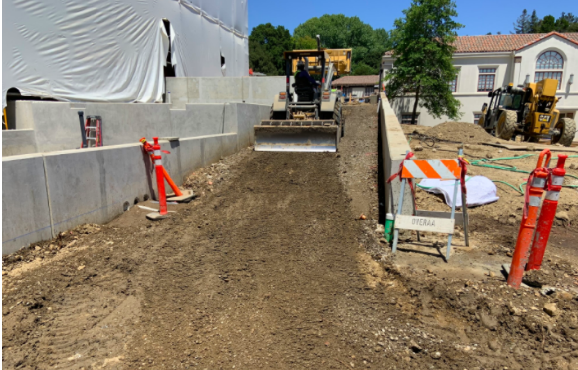
Construction of the pedestrian ramp and retaining wall between the STEAM building and Quad.
